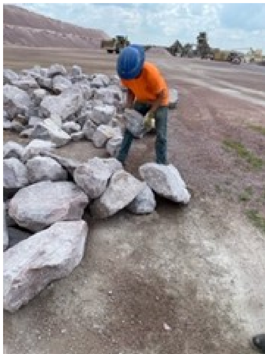
Hand Picking smaller size of riprap
